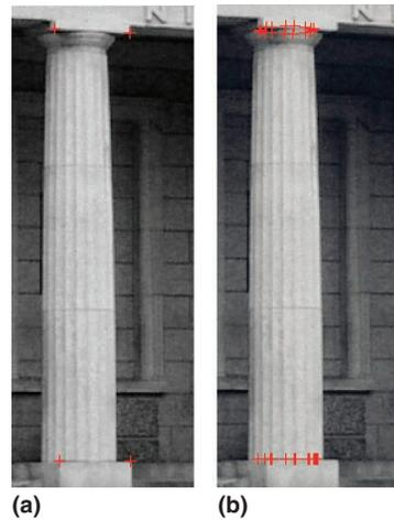
**4 The system (a) extracts four seed points on the base and crown, then (b) automatically adds column points.**
